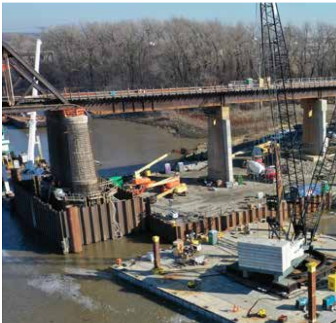
Constructing the bridge pilings
